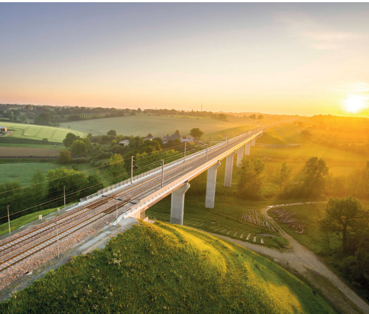
The Vicoin viaduct at Saint-Berthevin (France) on the Bretagne-Pays de la Loire high-speed rail line that Eiffage will operate until 2036.
