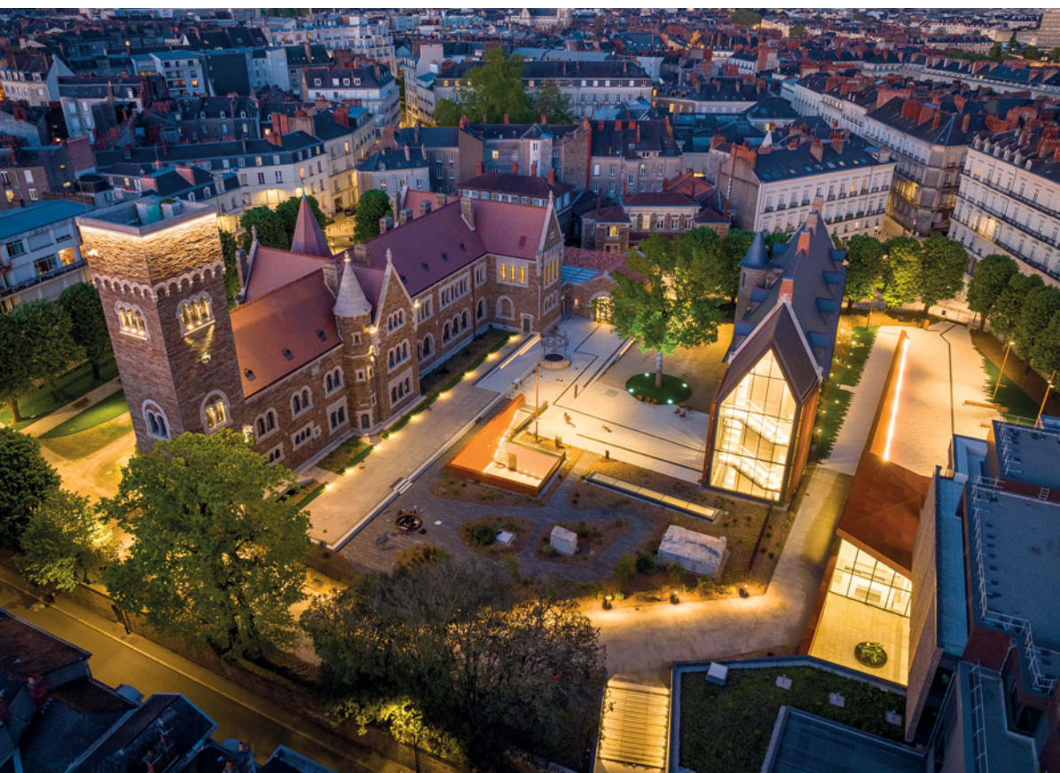
Illumination of the Dobrée museum in Nantes by Eiffage Énergie Systèmes' teams.
